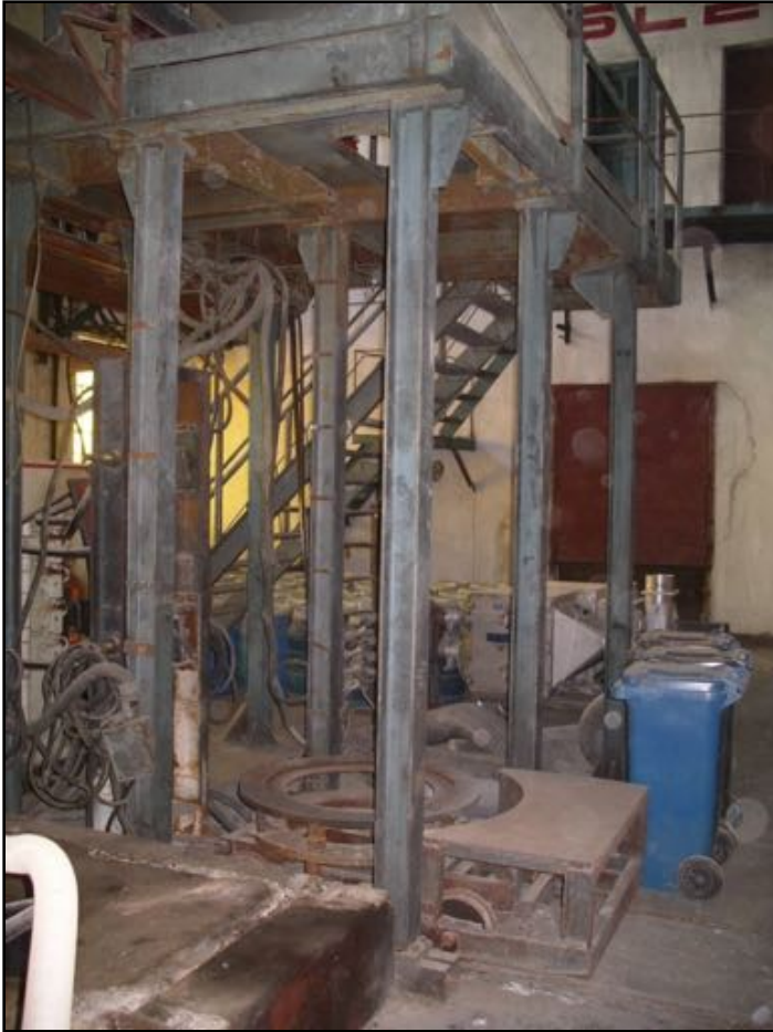
Bldg. 4 after disablement of a casting furnace
