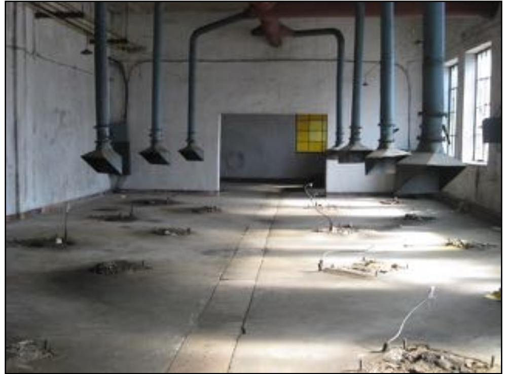
Bldg. 4 after removal of lathes
