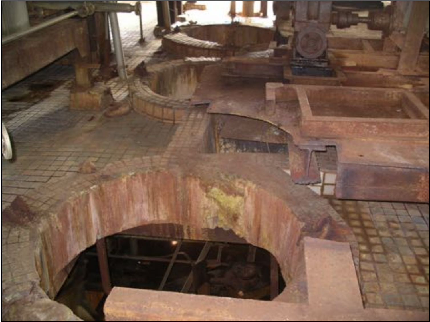
163 (Building 1: Fuel fabrication facility)
