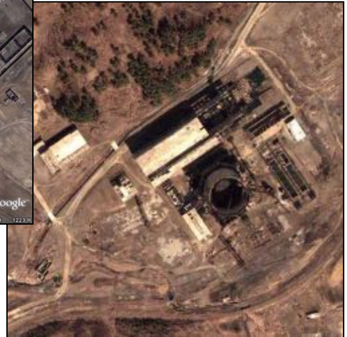
200 MWe reactor Taechon Construction site. Not salvageable
