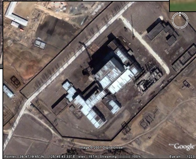
50 MWe reactor Construction site. Not salvageable
