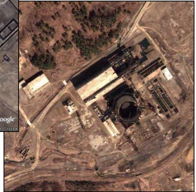
200 MWe reactor Taechon Construction site. Not salvageable
