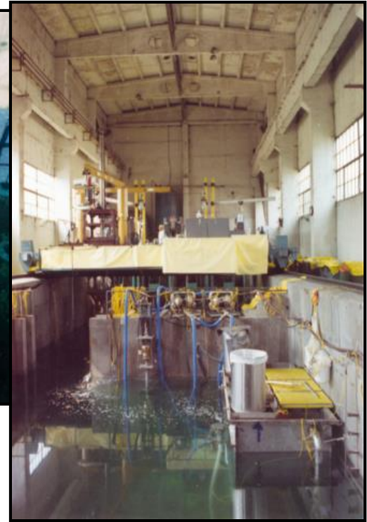
Spent fuel building (during canning team effort)
