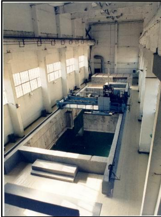
Spent fuel pool building (before)
