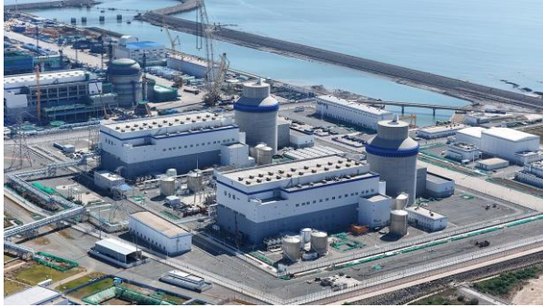
Haiyang Nuclear Power Plant units 1 and 2, 2024 · WPTO
