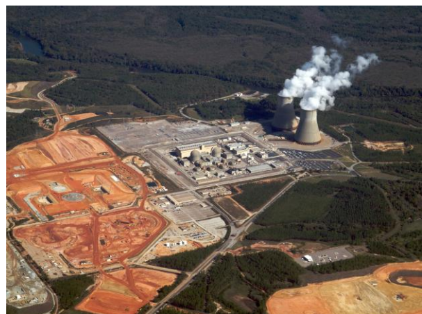
Vogtle plant with the future units 3 and 4 construction site at left, 2011 · Charles C. Watson Jr.
