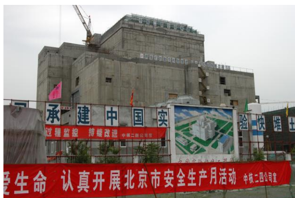
China Experimental Fast Reactor under construction, 2004 · Petr Pavlicek / IAEA
