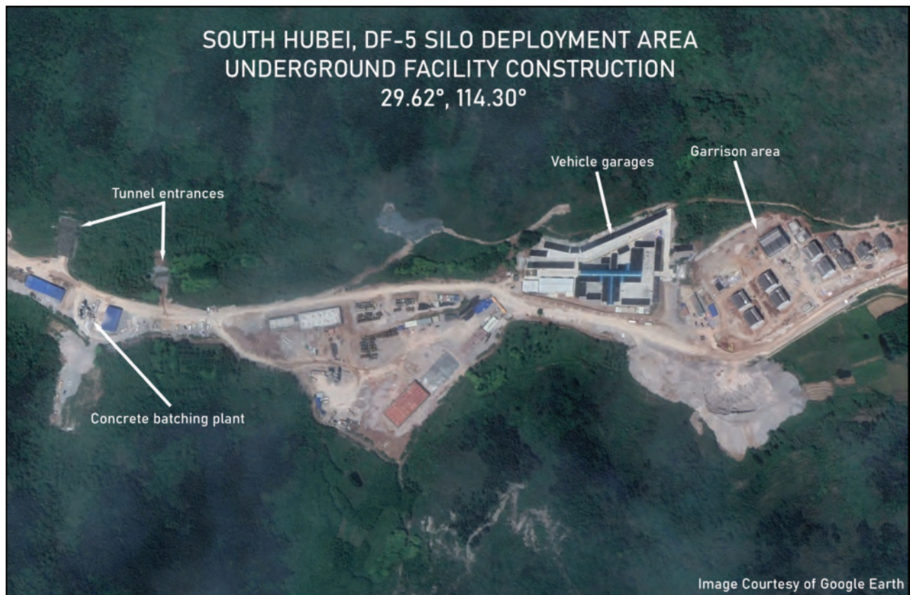
An underground facility under construction at PLARF Brigade 96734. Google Earth .
