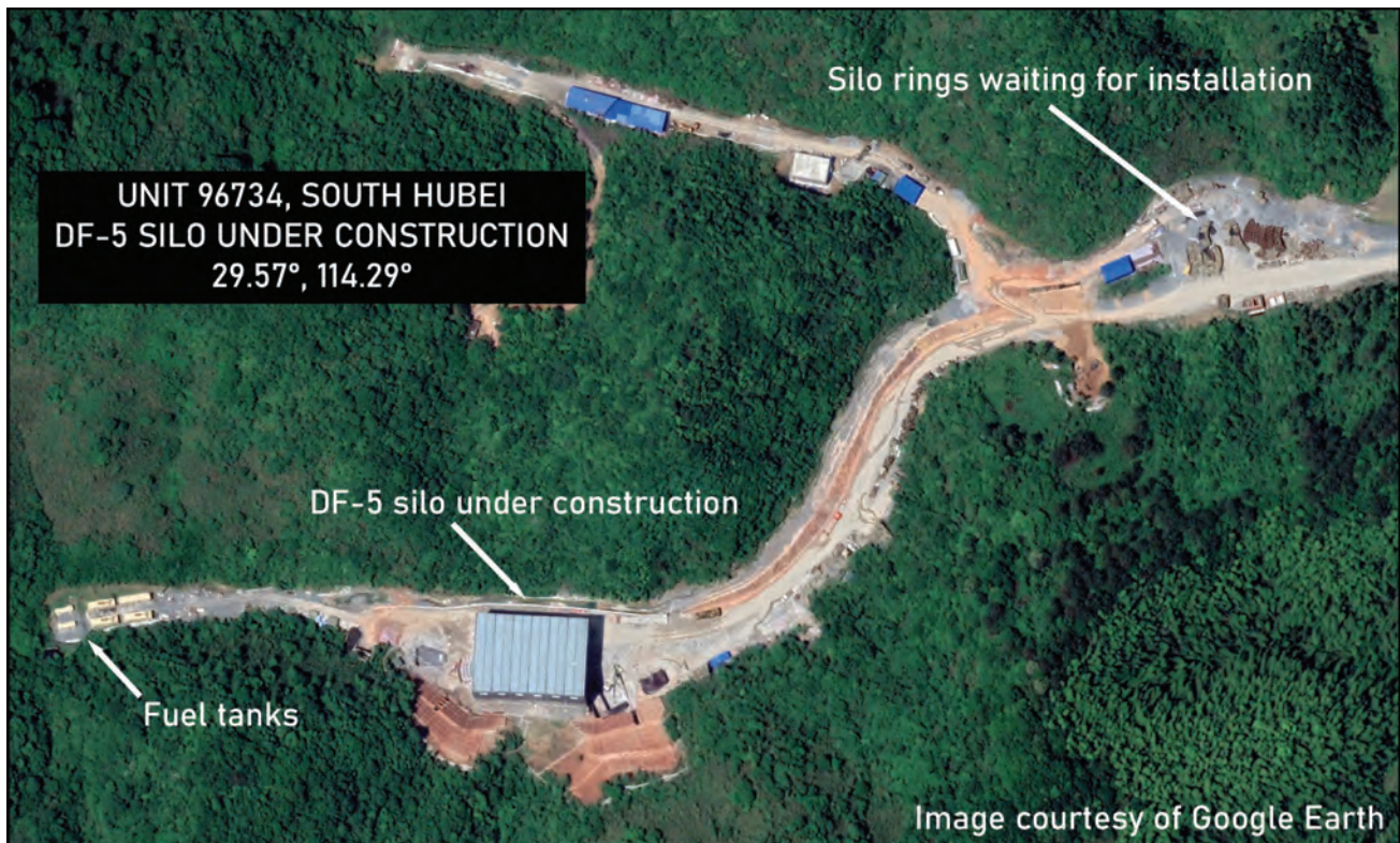
A DF-5 pattern silo under construction at PLARF Brigade 96734. Google Earth.
