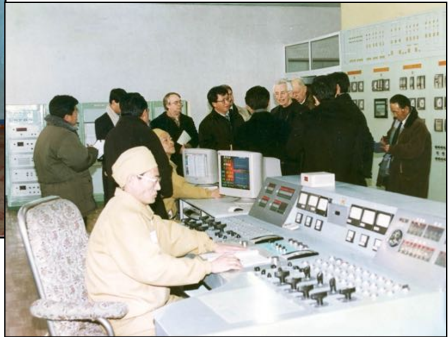
Reactor control room
