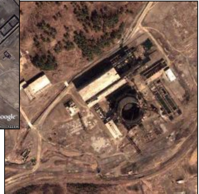
200 MWe reactor Taechon Construction site. Not salvageable
