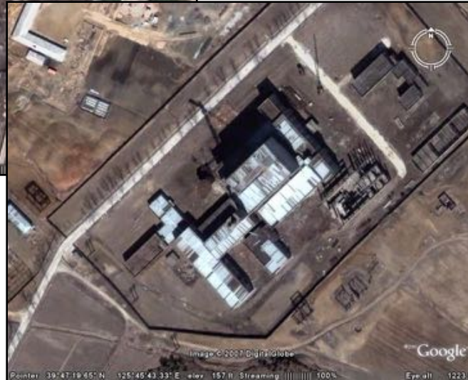
50 MWe reactor Construction site. Not salvageable
