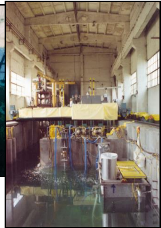
Spent fuel building (during canning team effort)
