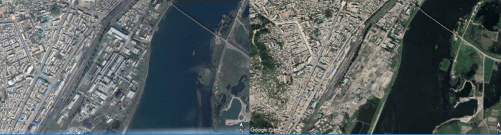
Images from Maxar via Google Earth from April 22, 2017 (left) and August 31, 2018 (right) showing the deconstruction of the old structures at the site of the new Sunch'on Phosphatic Fertilizer Factory.
